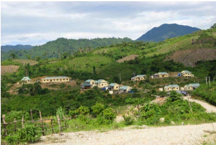
Figure 4: New housing in the Sông Tranh 2 re-settlement area
